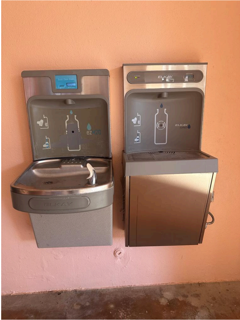
Water fountain station has an area dedicated to refilling aluminum water bottles. This decreases the number of plastic bottles used and incentivizes students to bring their own water bottles.
