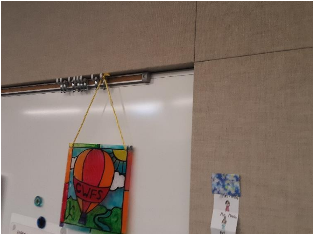
Figure 6 Engineered Acoustic Treatments Reduce Classroom Noise
