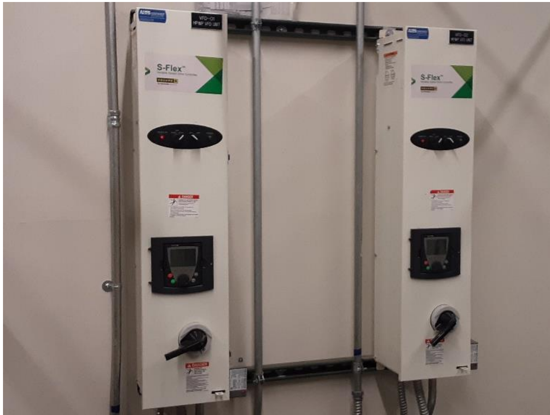
Figure 2 Variable Frequency Drives on HVAC Pumps Dramatically Reduce Pumping Energy Use
