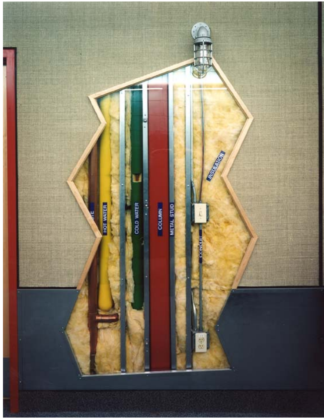
Cutout showing hot and cold water pipes, columns, metal studs, conduits and insulation within the walls at Bacon Elementary.
