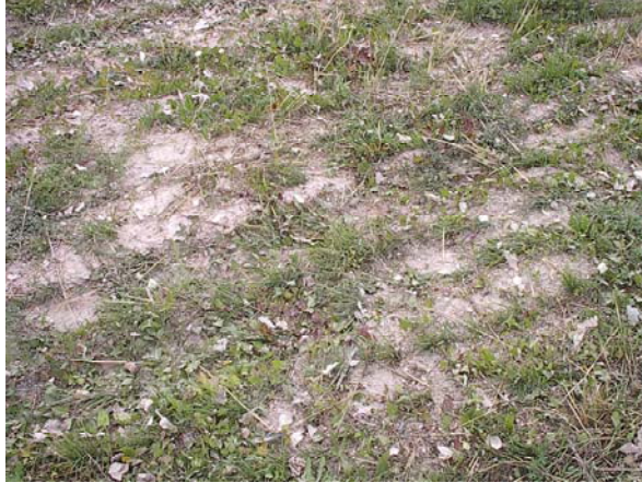
Ground drywall spread across the future site of Fossil Ridge High School.
